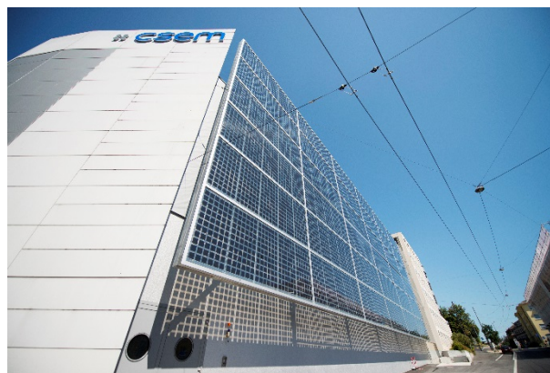
Figure 2: Solar façade on the CSEM building in Neuchâtel.
